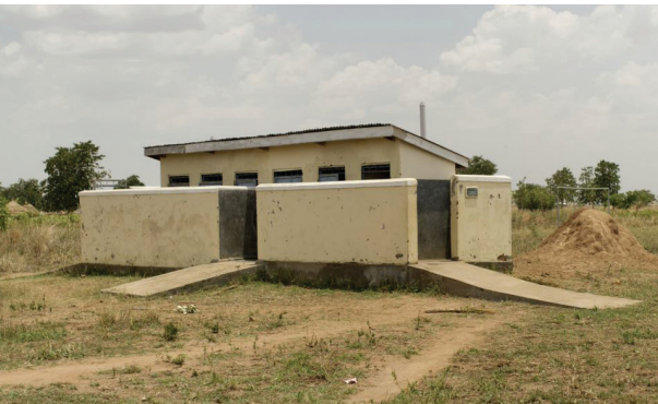
The new toilet facilities at Pacaka Primary School
